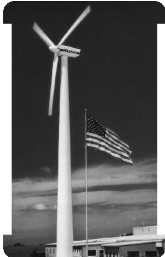
Wind turbines, such as this 225-kW machine in Adair, Iowa, could play a role in the nation's expanding market for distributed generation. The turbine shown here provides electricity for Schaefer Systems, Inc., a plastics manufacturer. Photo courtesy of Vestas - American Wind Technology, Inc.
