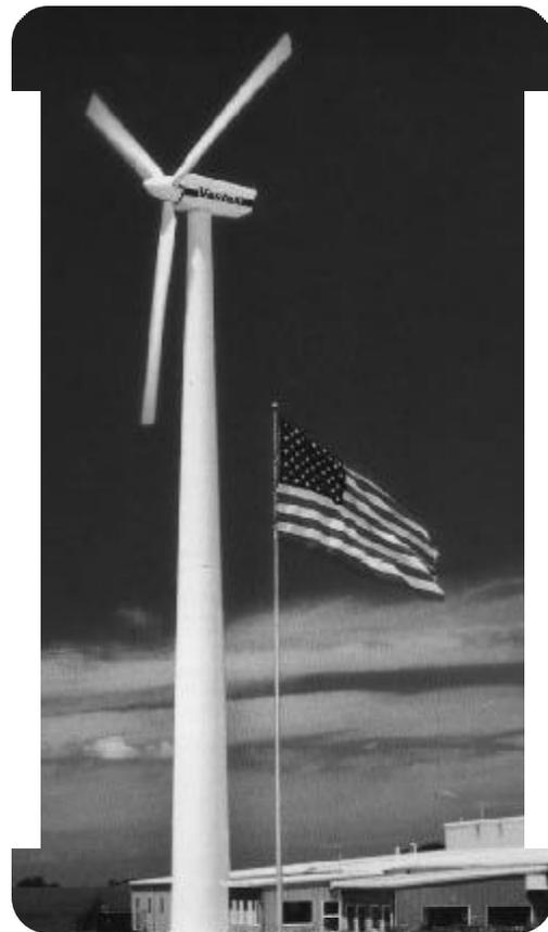
Figure: 1.1 Schaefer Systems 225-kW Turbine. Wind turbines, such as this 225-kW machine in Adair, Iowa, could play a role in the nation's expanding market for distributed generation. The turbine shown here provides electricity for Schaefer Systems, Inc., a plastics manufacturer. Photo courtesy of Vestas - American Wind Technology, Inc.
