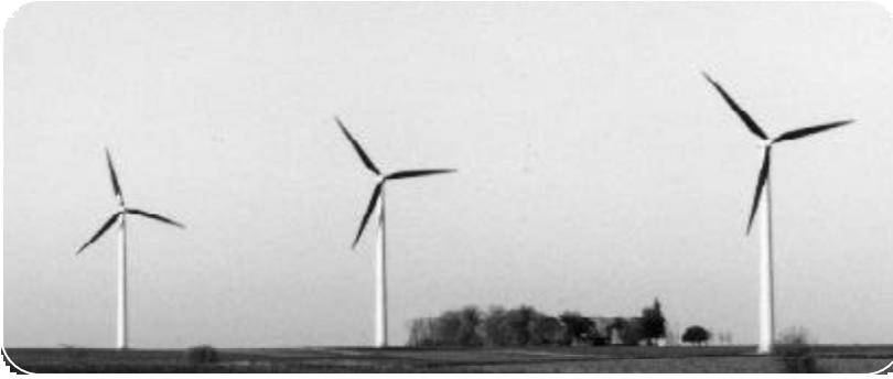
Figure 3.4 Iowa Joint Municipal Utility Project 3 x 750 kW. As part of the 2.25-MW Iowa Distributed Wind Generation Project, researchers are testing the ability of advanced turbine technology to minimize power quality problems on a weak distribution system. Photo courtesy of Thomas A. Wind.
