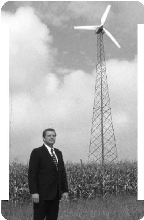
Figure 3.2 Waverly Light and Power 80-kW turbine shown here with Waverly's Manager Glen Cannon, who championed the project. Waverly Light and Power's 80-kW Zond Z16 turbine was the first in Iowa to be utility owned and operated. The utility's success in demonstrating the technical feasibility of interconnecting distributed wind generation led to a new 2.25-MW project in Algona that is owned and operated by seven Iowa municipal utilities. Photo courtesy of Ken Formanek.
