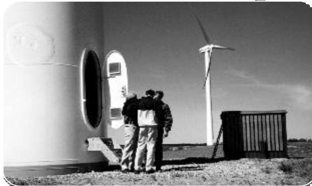
Figure 3.5 Turbine and typical electrical equipment enclosure on a Danish farm. Like other turbine owners, Gravers Kægaard was responsible for providing electrical facilities for interconnection. He built the enclosure on the right to house a circuit breaker, step-up transformer, fuses, and meters for a three-turbine cluster. Kægaard uses the door on the left to gain access to electrical controls and a ladder inside the turbine tower. Photo courtesy of Thomas A. Wind.
